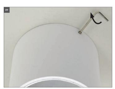
**09** Tighten grub screws with Allen wrench on both sides. Check the luminaire for tightness.
