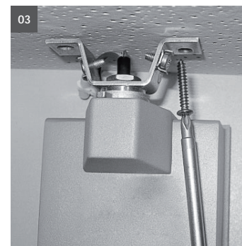
03. Strahler montieren 03. fix the spotlight at the ceiling
