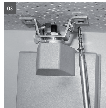
03. Strahler montieren 03. fix the spotlight at the ceiling
